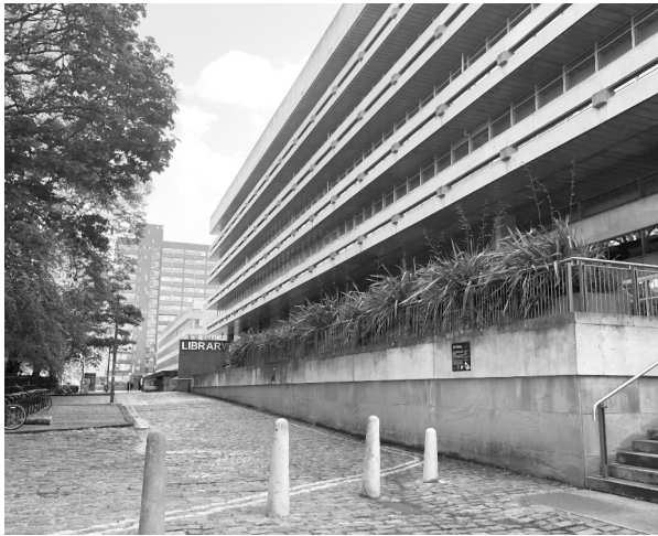
Fig. 2: George Square south, Edinburgh, showing Matthew's Arts Tower and departmental buildings (background) and Spence's University Library (right foreground), photo 2020
