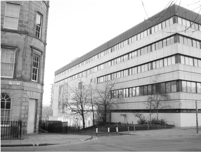
Fig. 1: Edinburgh Royal Infirmary Redevelopment, 'Phase One', photo 2017. Temporary walling (left) shows where later phases would have adjoined
