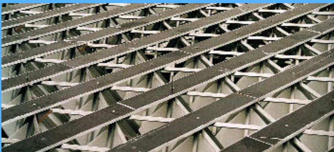
Boards of birch plywood are fixed with bolts to the node points of the construction. The boards are treated against dampness with epoxy and light primer.
