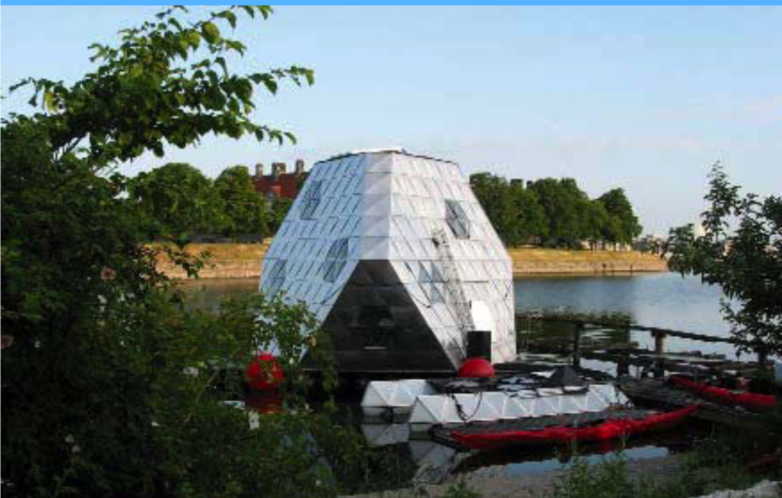
FLOATING PLATFORM, N55 SPACEFRAME and MODULAR BOAT, 2002. The batteries for the boat engine are charged by the solar panels on the roof of N55 SPACEFRAME.
