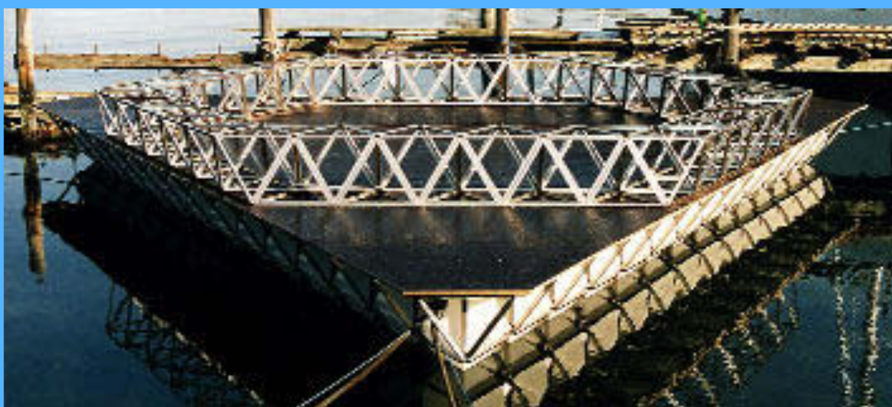
The top construction is fixed directly onto the wood as well as with bolts through the wood to the platform.
