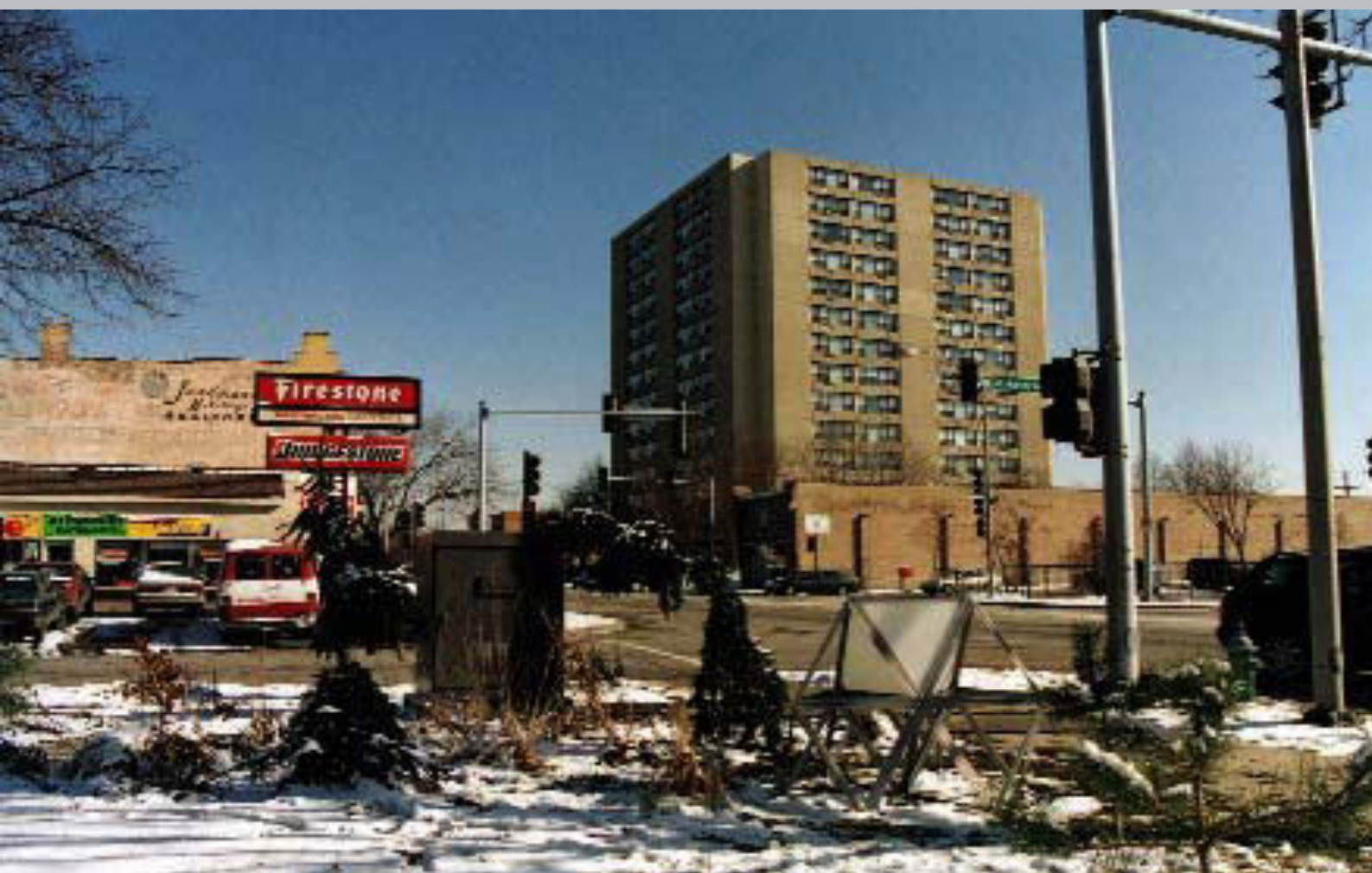
Position: N 41° 53' 03,4" E 087° 46' 06,8". Area: 160 m 2 . Chicago, USA.
