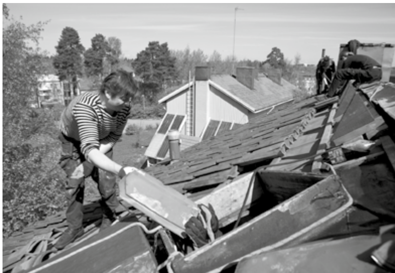
Work on the houses is done by the tenants themselves © Laura Böök
