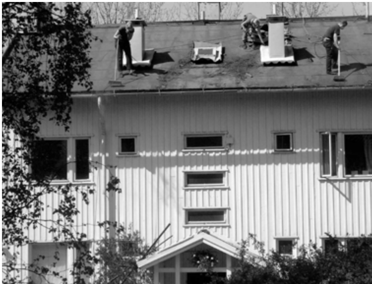
Renovating a roof the Oranssi way © Anu Brask
