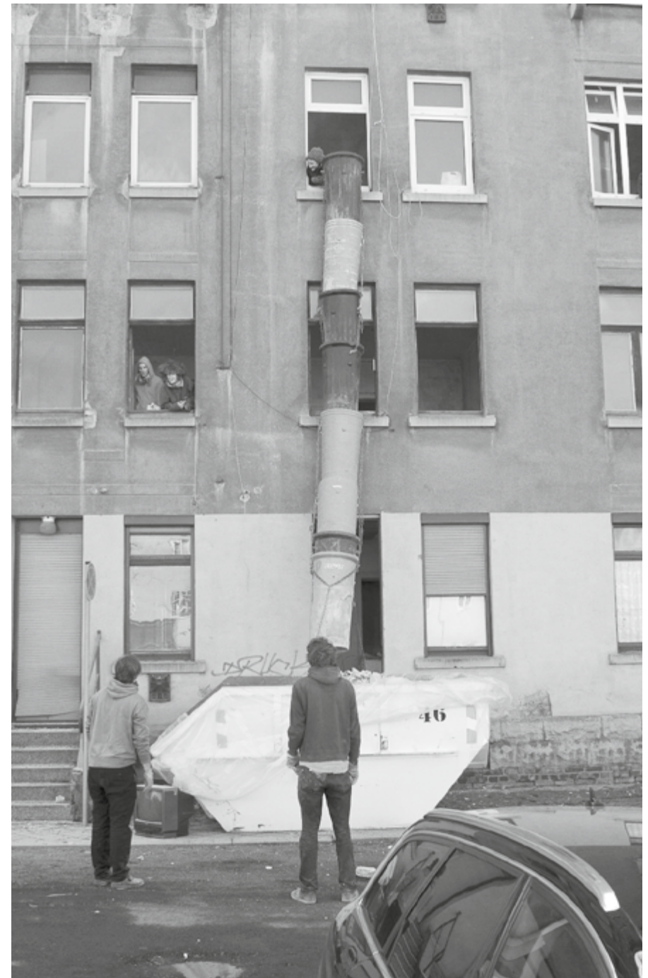
Renovating together © Paul Ruben Mundthal
