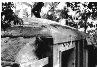
Lightweight concrete on.
