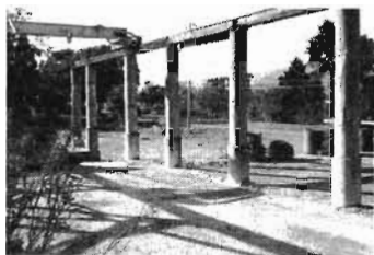
Box columns made from concrete sewer pipe, filled with concrete.
