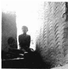
Cow dung plaster in an Indian village house.
