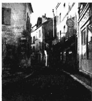
Slight angles in the building fronts.
