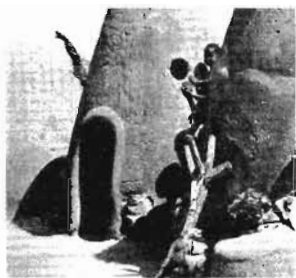
A door frame as a thickening.
